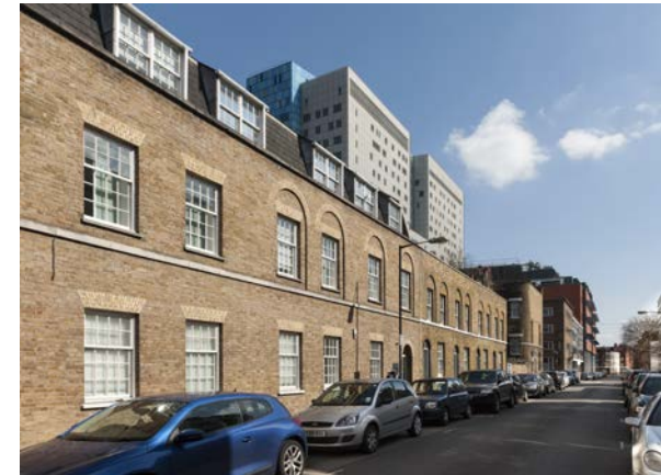
Yvonne Carter Building, Ashfield Street.
