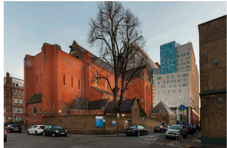
St Philip's Church, view from Newark Street looking north-east.
